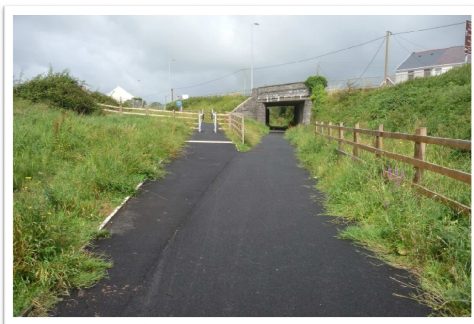
Photo above: Improvements to walking and cycling facilities in Carmarthen
